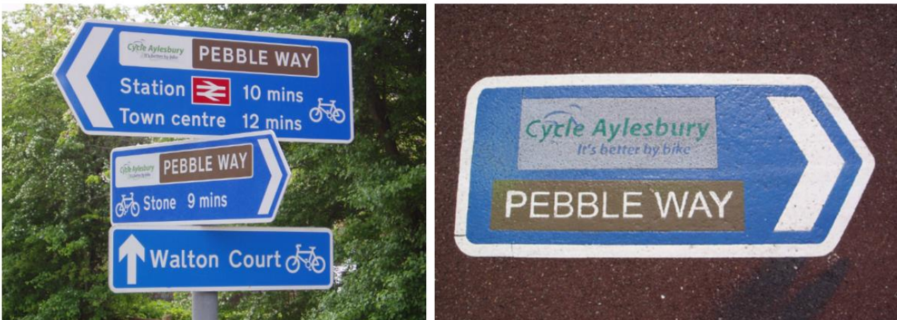
Figure 7-14: Left: Signing in Aylesbury showing route branding and local destination off the main route. Right: Thermoplastic marking used only off-highway
